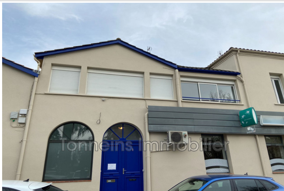
Office 3720TI Tonneins
