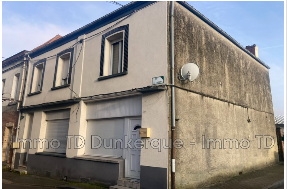
Building TD44 Bruay-la-Buissière
