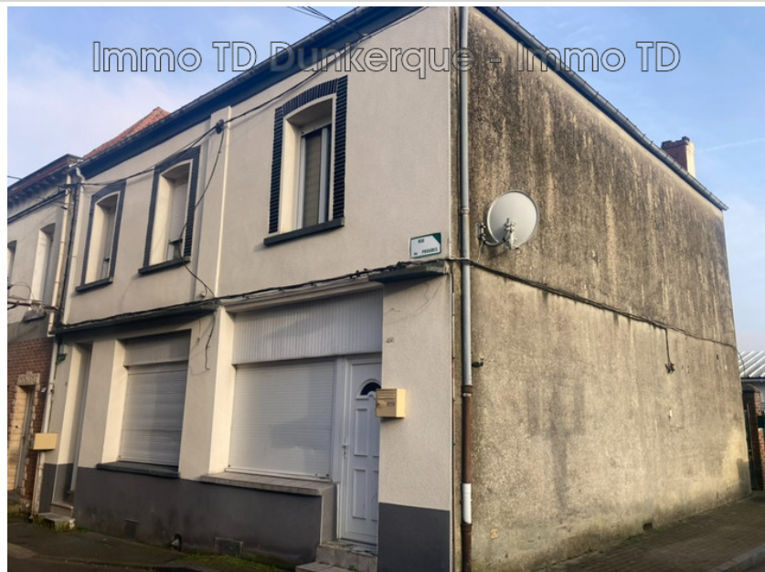
Building TD44 Bruay-la-Buissière
