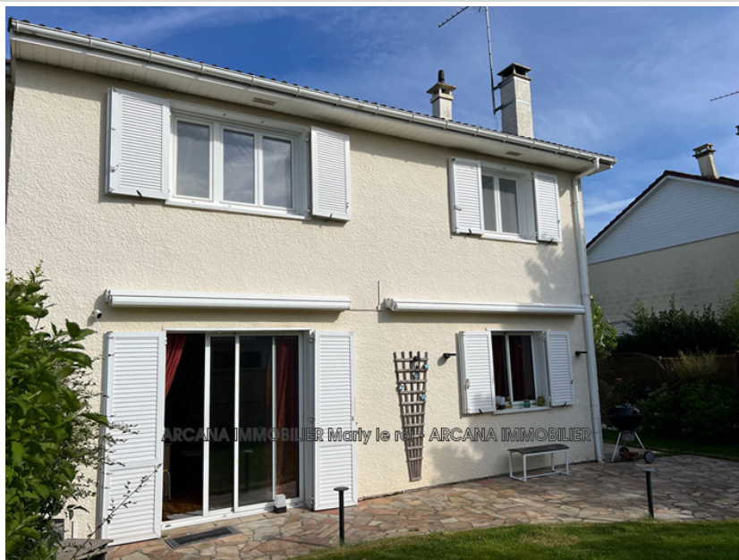
House 1507A Mareil-sur-Mauldre
