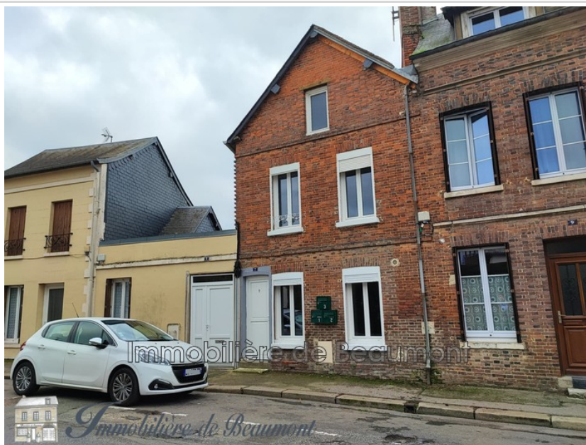
Building 486 Le Neubourg
